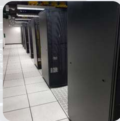
Double floor, raised floor to prevent water leakage that may cause damage to computer equipment
